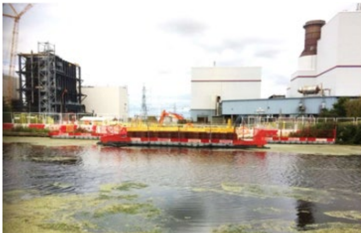
Plate NTS9: Typical cofferdam that would be required on the canal, adjacent to the intake for Keadby 2 Power Station
